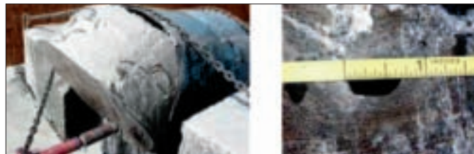
Fig. 2. Cracked cement annulus after acid-soluble test (left), and perforation hole diameter on the 6.625" casing (right).
