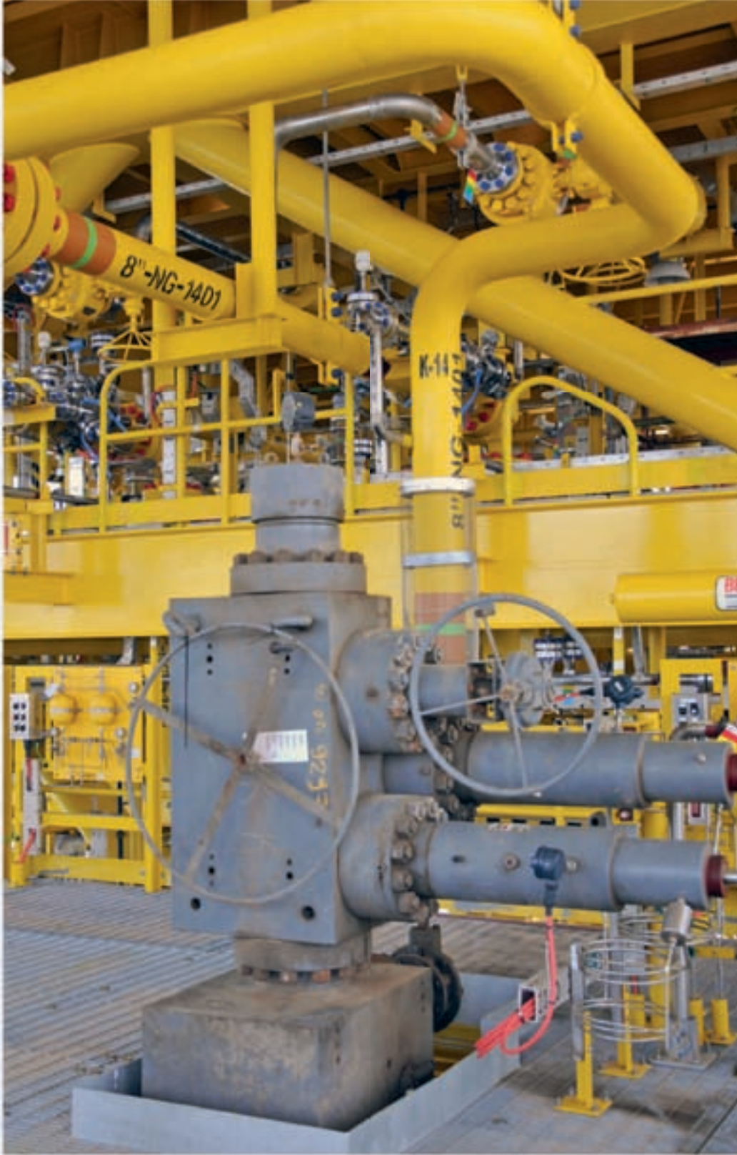
A wellhead in the Karan field. The valves and flow line control gas flow from the reservoir to the surface and into the trunk line that carries natural gas to the gas plant for processing into the Master Gas System and distribution to the customers.
